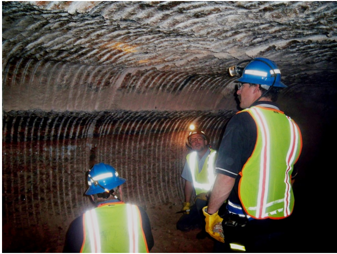
Mining Safety Board members inspect back and wall conditions at Intrepid Potash underground mine near Carlsbad, NM
