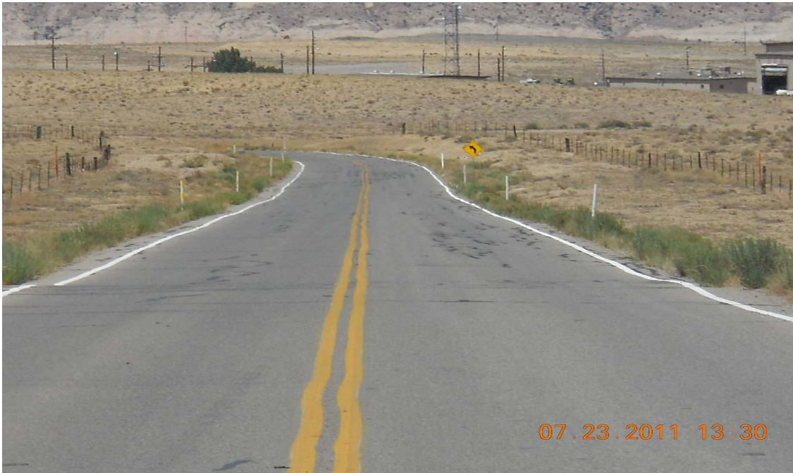
Access Road to Navajo Mine that was the location of the only mine fatality during 2011 in New Mexico
