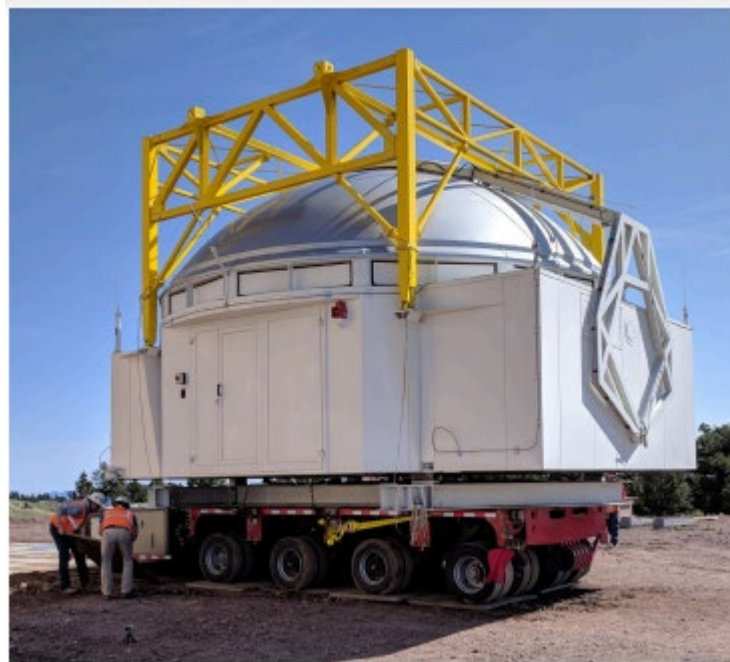
Figure 3: UT installed on transporter/jig.
