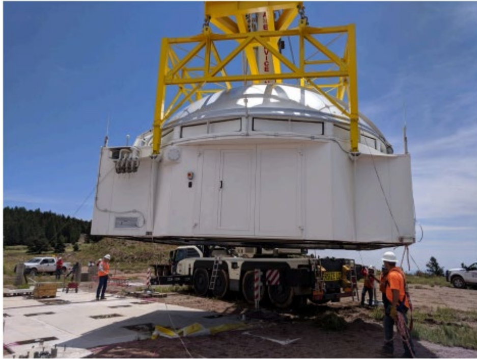
Figure 4: UT being installed on array pad.
