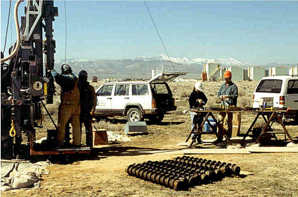
**Figure 5-6.** Hollow-stem auger drilling and sample collection of vadose zone core, UE6s, at Yucca Flat, Nevada Test Site.
