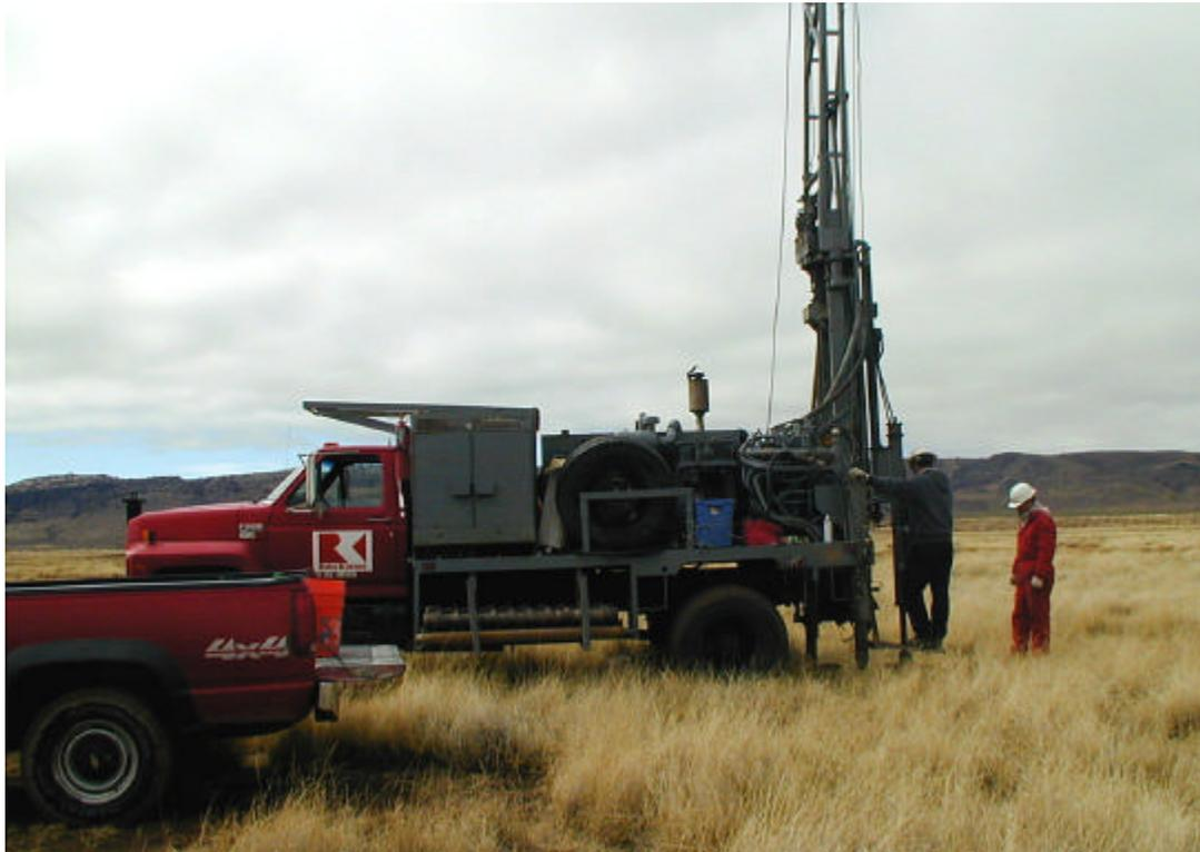
**Figure 6-8.** Drilling using the hollow-stem augering method. Photo taken at the Miller Ranch grassland site, drilling borehole designated as GD.
