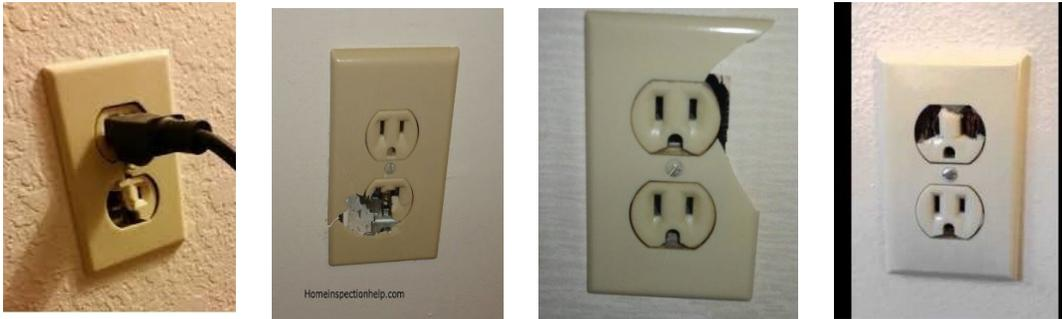
Even if only one outlet appears to be affected it is unsafe to use the entire outlet. Foreign objects, dust and debris can get into the outlet and potentially create an arc—a continuous electrical current that develops so much heat from the charge carrying ions or electrons that it can vaporize or melt anything within the range of the arc.
