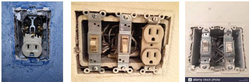
Loose and missing covers put you at risk of coming into contact of a live wire and increase the probability of an arc from dust and debris.
