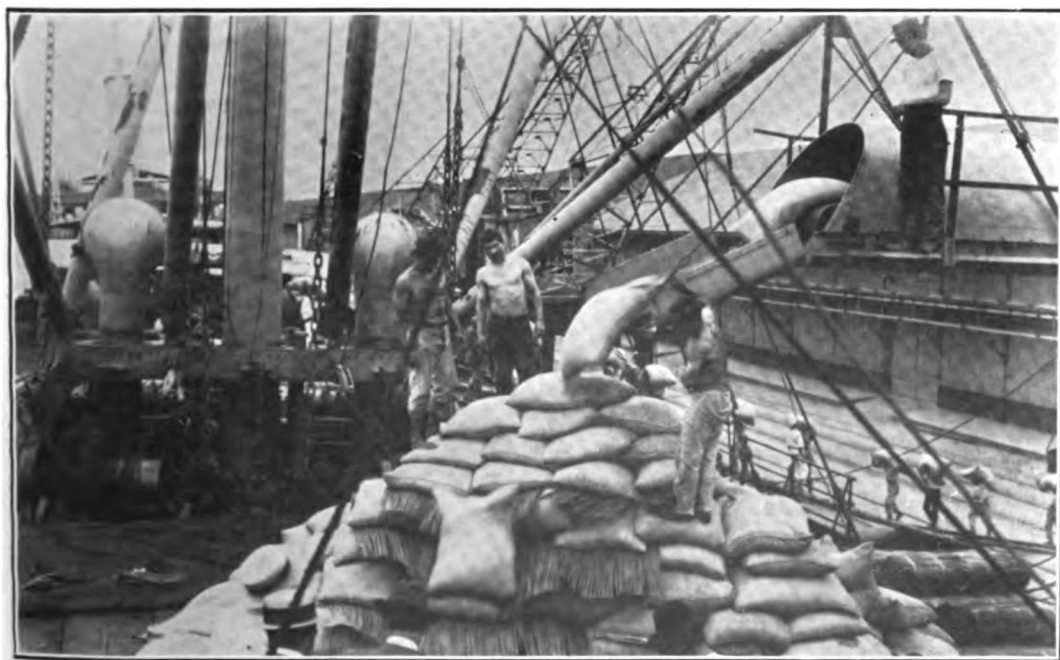
HERE THE AUTOMATIC BELT POURS INTO THE HOLD A CONTINUOUS STREAM OF BAGS OF COFFEE OLD AND NEW METHODS OF LOADING COFFEE AT SANTOS
