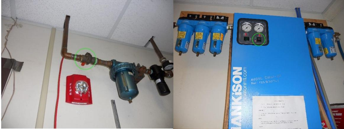
The gas is pictured on the left, turn the perpendicular red handle to the open position such that it is parallel with the pipe. On the right is the Blue Hankison unit, flip the rightmost switch to the on position. Order is crucial in this step to prevent damage to the instrument.
